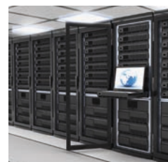
NTP Time Server
